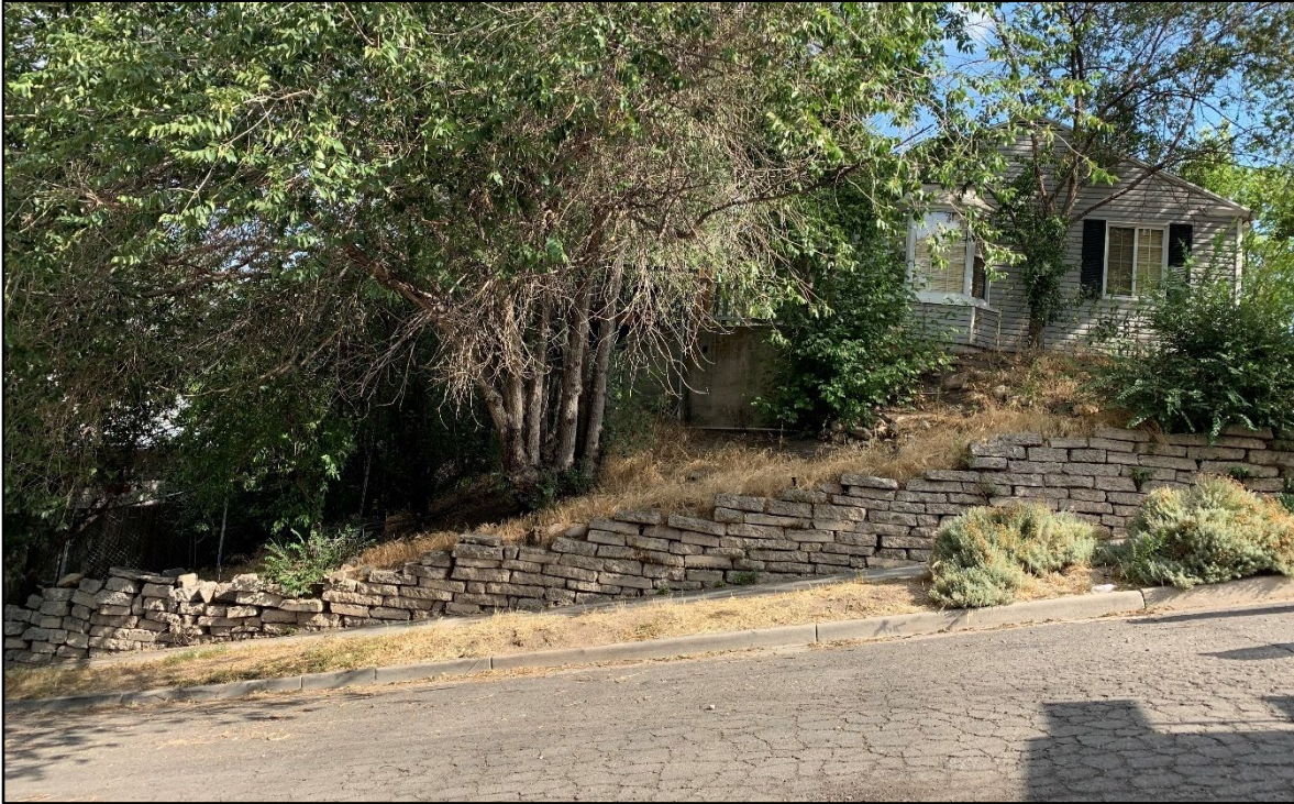
Southern property line along Harrison Avenue – Looking north
