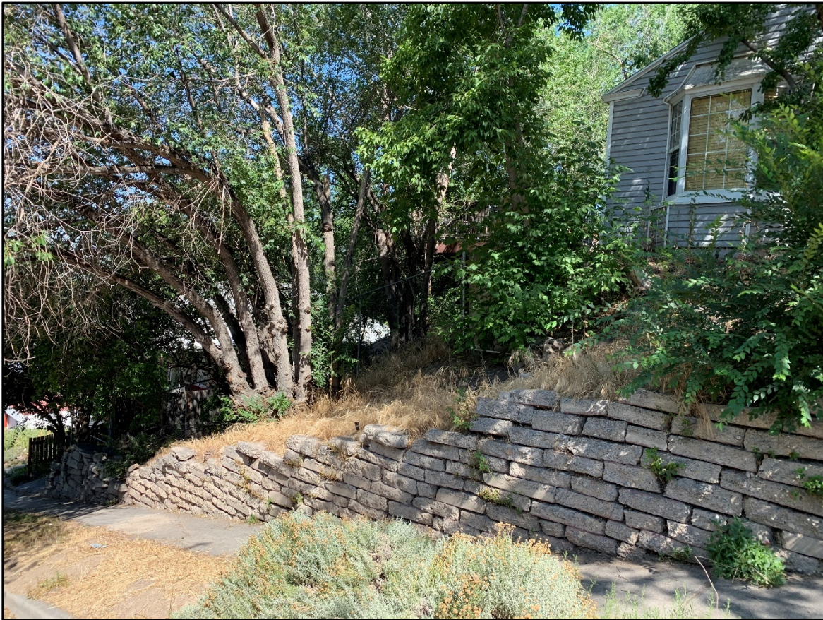
Existing retaining wall
