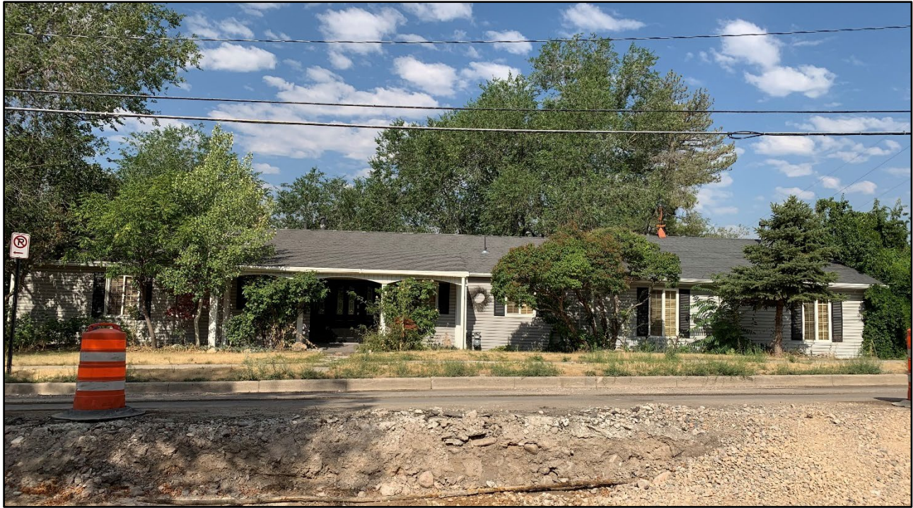
Existing Dwelling Unit – 1362 S 1300 E
